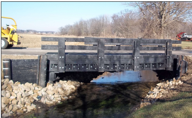
Bridge 174-0.56 over the Onion Ditch
